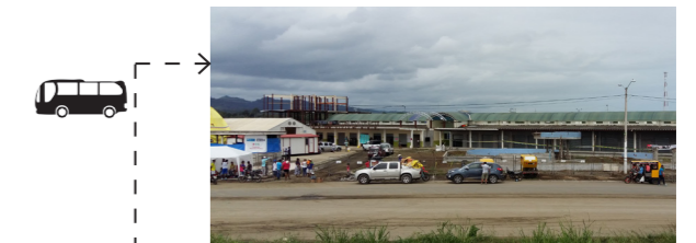
Figura 10. Terminal terrestre Autor: Juncay 2016
