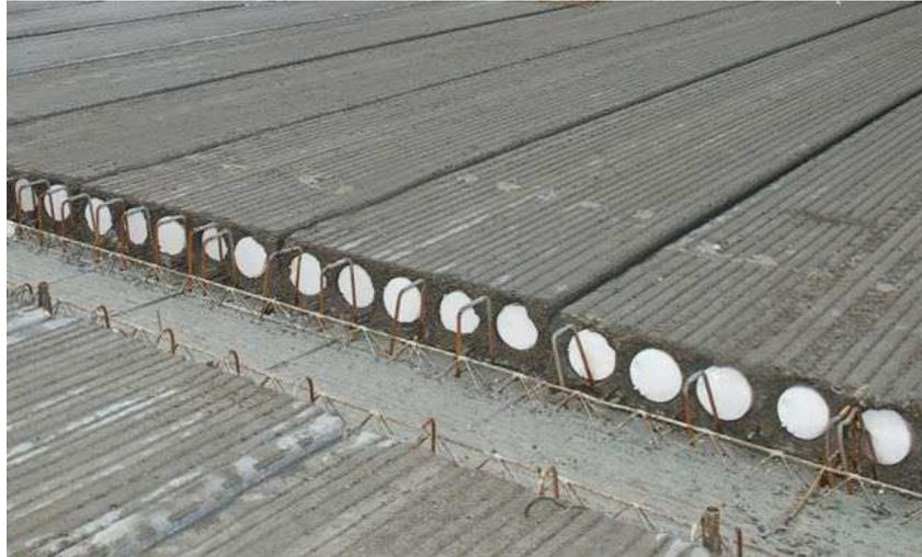
Fig. #34 Losa pretensada (A fine WordPress.com site, 2013)
