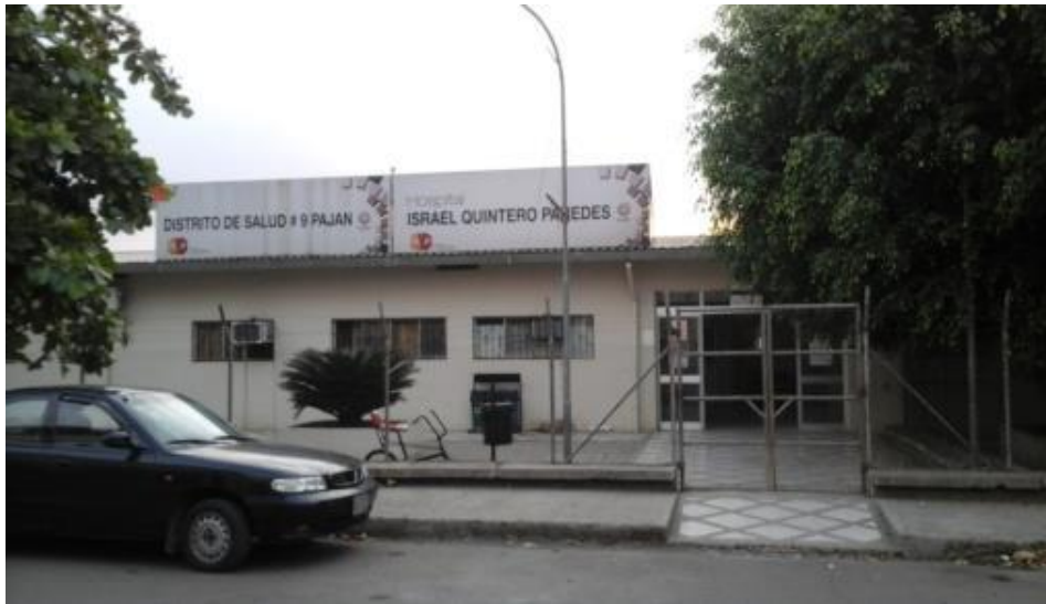
Figura 2: ingreso principal del Hospital
