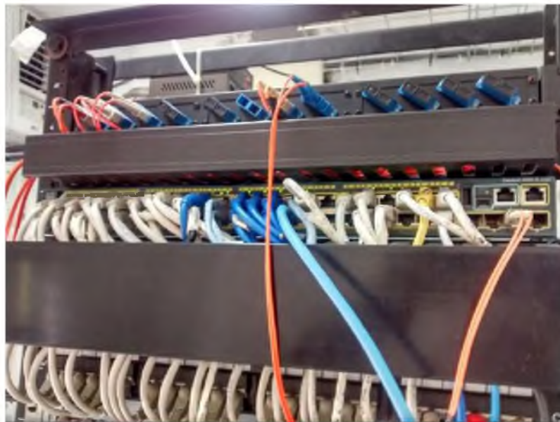
Figura 4. 3: Switch Cisco Catalyst 2950 del rack principal bloque administrativo
