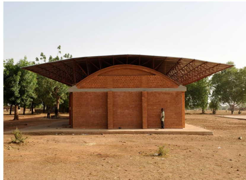
Figura: Gando Primary School de Kéré Architecture Fuente: ArchDaily.
