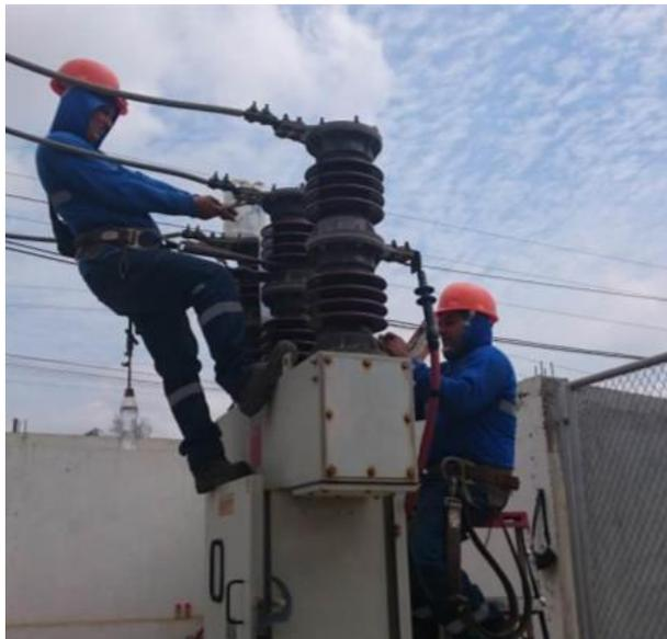
Figura 4. 4 Interruptor de 13.8 KV
