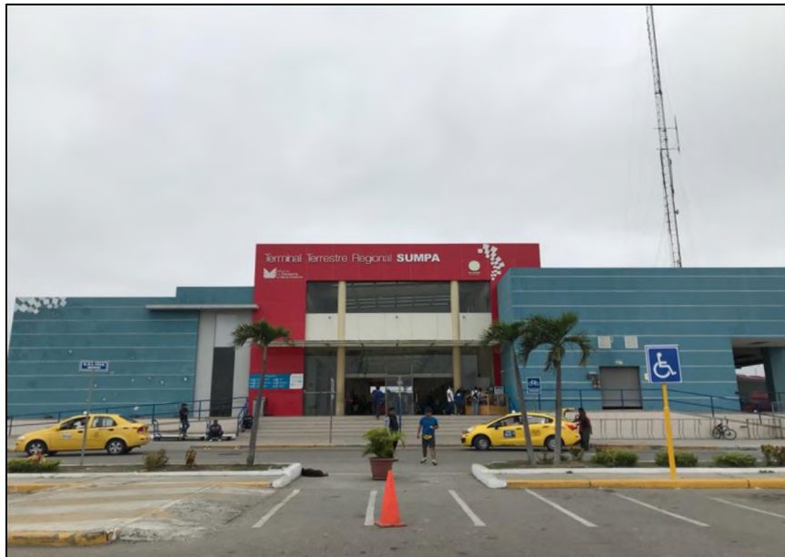
Figura 3. Terminal Terrestre Regional Sumpa
